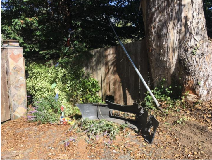
Figure 2. Bumper and skid marks in driveway of 446 Panoramic after car ricocheted off 455 Panoramic Hwy. entryway wall, lost control, crossed Panoramic Hwy. hit eucalyptus tree 446 Driveway entrance, took out tree, posts, and fence and car was totaled.
